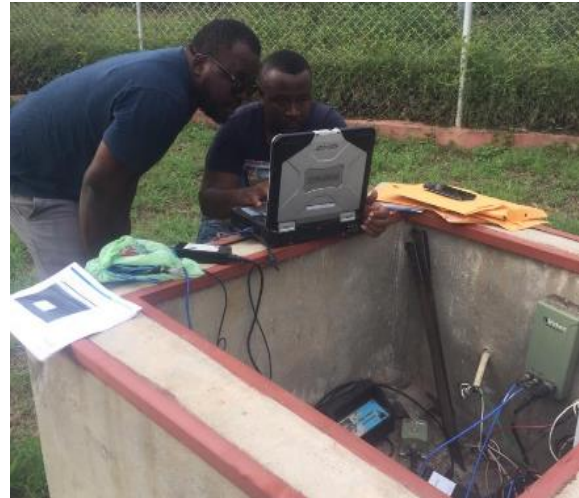
Project's RDM expert and UTS's technician repairing the seismology station in Cap-Haïtien, November 2019
