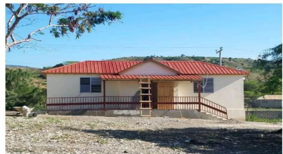
Construction of a dormitory and of a warehouse at the COUD of the North-west, 2019
